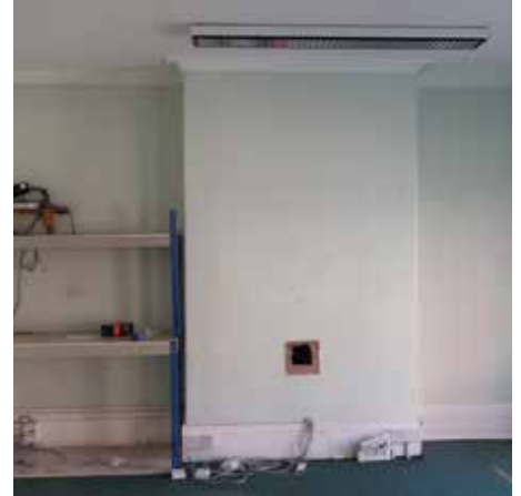
(v) Chimney breast
