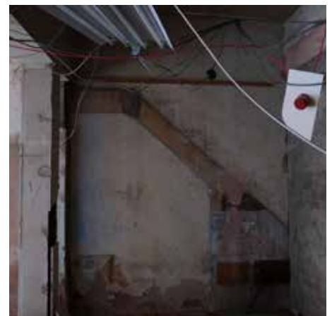
Evidence of past staircase (Ground Floor)
