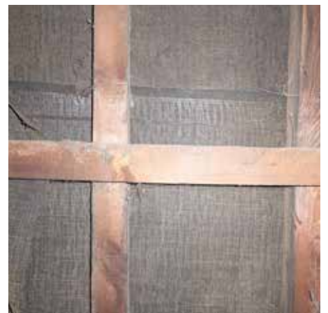
(xii) New roof timber/ felt
